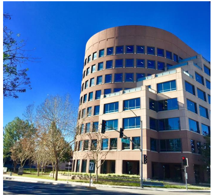
This is the Caltrans District 12 Building in Santa Ana. (Photo Credit: Caltrans District 12)
